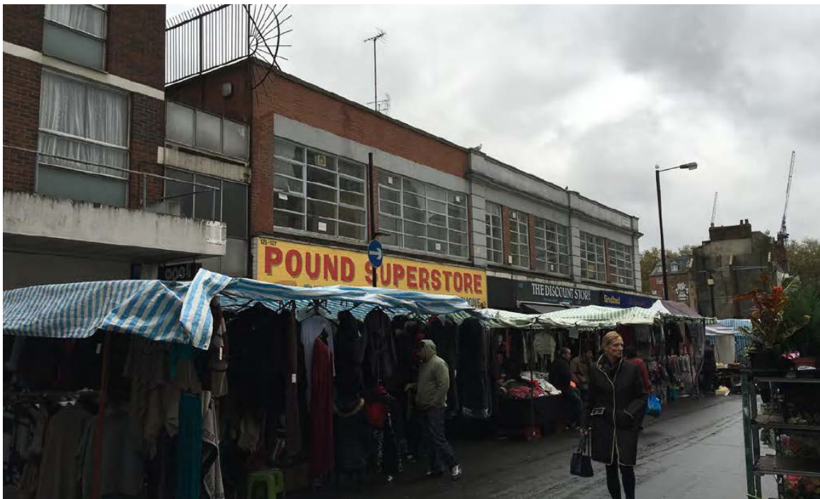
Application site as seen from Church Street.
